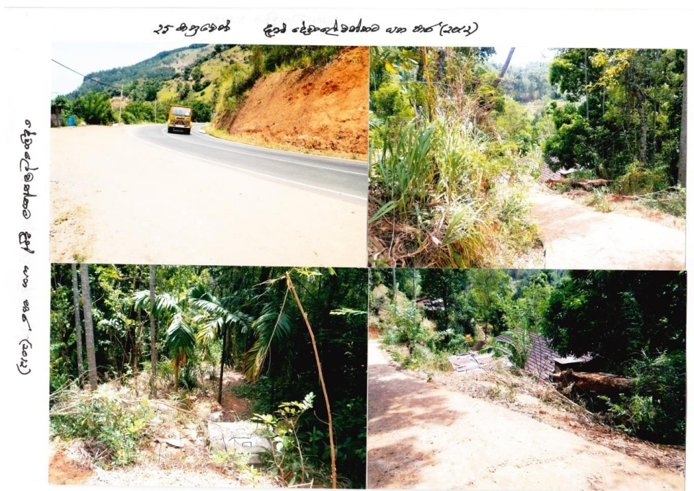
ROAD TO DEWALEWATHTHA FROM THE MAIN ROAD 25 TH MILE POST.
